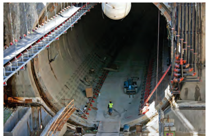
A section of the tunnel excavated by Bertha
